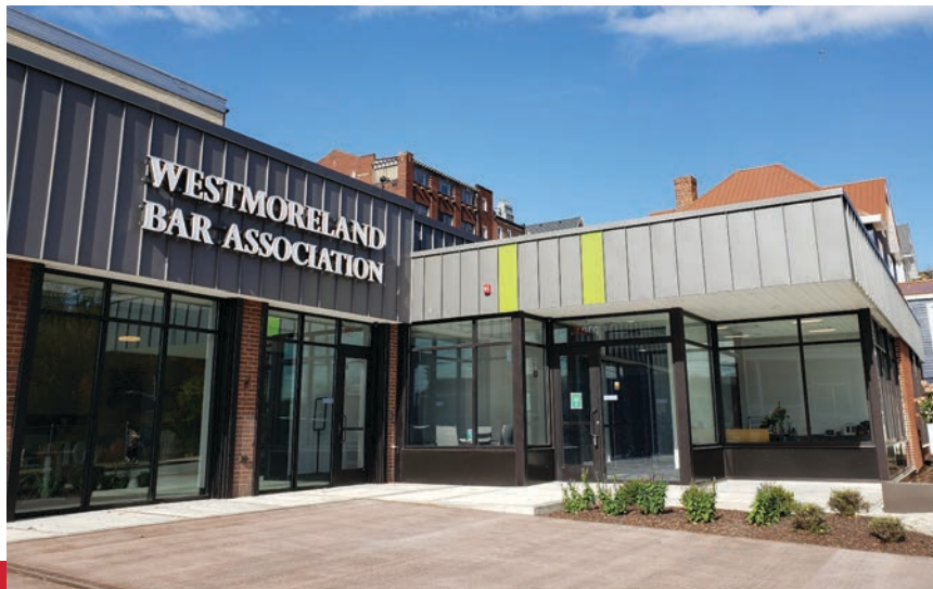
The new headquarters of the Westmoreland Bar Association, located at 100 North Maple Avenue in Greensburg.
